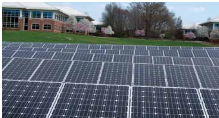
Solar panels, here at the George Washington Carver Center in Beltsville, Md., may help the U.S. bid fossil fuels farewell.
